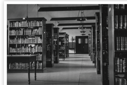
Original Second Floor Library
